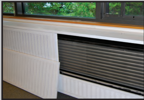
Bridgewater State University Bridgewater, Massachusetts LEED® Silver
