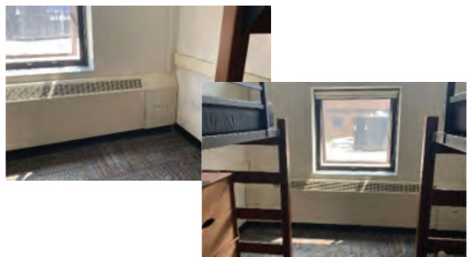
Example of housed fin tube, radiant heat elements
