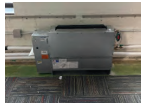
Example of a typical FCU, no factory housing option
