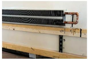
f.) Connect the Supply and Return piping to complete the circuit. If using a BUC, it will be necessary to install the BUC first before the main Supply and Return piping is ran and connected.
