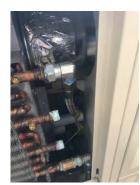
b.) The vertical chilled/hot water pipes are connected via flexible hoses that run through a pipe work knockout on the top or side of the unit.
