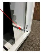
d.) If inspection of the Fin Tube Elements is needed, remove the Rear Fin Tube Element Grill on the back of the QLCI. Locate the (2) socket head screws on the top of each Rear Fin Tube Element Grill. Loosen the locking screws using a 5/32" Allen Wrench and remove the QLCI Rear Fin Tube Element Grill as shown below. Make sure when placing the QLCI Rear Fin Tube Element Grill back in place that the side tabs interlock with the metal flanges.
