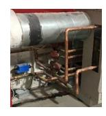
c.) Piping should be insulated and properly labeled in accordance with local building codes as shown below.
