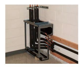
b.) Install threaded ½" NPT connections (provided by others) on each pipe or solder straight end connections 2" to 3" from the point where the QLCI units connect to each other along the wall as shown below.
