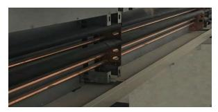
f.) Alternative piping method 2: QLCI units can allow the piping runs to be in the front of the units above the hydronic coil. This allows the QLCI to be mounted to the 2x4's first, then connect the ductwork before making the piping connections. The feeding pipework can be routed through the side wall knockouts. QLCI's and piping connections can be connected in the front as shown below.
