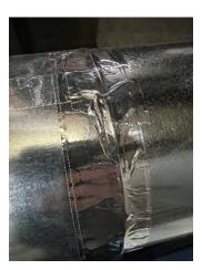
Ensure there is an airtight connection between the supply duct and each QLCI duct interconnections. Duct connections should meet SMACNA class B standard up to 2 in. W.G. Refer to Division 23 – Heating, Ventilation and Air Conditioning (HVAC) Section 23 31 13.01 "Metal Ducts" and or Section 23 07 13 "Duct Insulation" for additional information.
