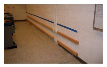
b.) The **2x4 Mounting Boards** should run the length of the QLCI installation (not individual units). The **2x4 Mounting Boards** should stop 1.5" from edge of wall to allow end unit side panel to set flush against the wall.
