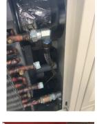
b.) The vertical chilled/hot water pipes are connected via flexible hoses that run through a pipe work knockout on the top or side of the unit.
