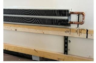
f.) Connect the Supply and Return piping to complete the circuit. If using a BUC, it will be necessary to install the BUC first before the main Supply and Return piping is ran and connected.
