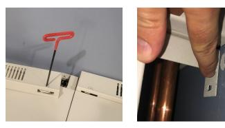
e.) Alternative piping method 1: Units can be placed on roller carts and connected to each other first. The pipework can be connected to the back of the QLCI's, and piping connections can be connected to each other before mounting the entire run of QLCI's to the wall mounted 2x4's as shown below.
