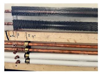
c.) Once all the piping is connected, test for leaks and insulate piping. Refer to project plans for insulation specifications. Use standard plumbing practices and test for leaks once the piping is complete. See **Section 4.1** for pressure ratings.
