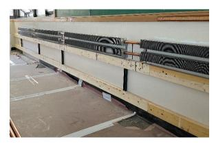
e.) Once all Fin Tube Elements are installed, begin joining all piping together (Straight pipe and fittings supplied by others). The lower Fin Tube Elements are to be the Supply run, and the upper Fin Tube Elements are to be the Return run. A Loop should be used to connect the last lower Fin Tube Element to the upper return row of Fin Tube Elements.
