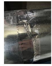
Ensure there is an airtight connection between the supply duct and each QLCI duct interconnections. Duct connections should meet SMACNA class B standard up to 2 in. W.G. Refer to Division 23 – Heating, Ventilation and Air Conditioning (HVAC) Section 23 31 13.01 "Metal Ducts" and or Section 23 07 13 "Duct Insulation" for additional information.
