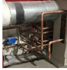
c.) Piping should be insulated and properly labeled in accordance with local building codes as shown below.
