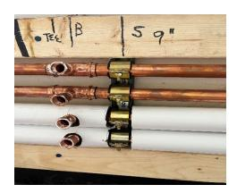
c.) Once all the piping is connected, test for leaks and insulate piping. Refer to project plans for insulation specifications. Use standard plumbing practices and test for leaks once the piping is complete. See **Section 4.1** for pressure ratings.
