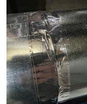
Ensure there is an airtight connection between the supply duct and each CB-SV duct connection. Duct connections should meet SMACNA class B standard up to 2 in. W.G. Refer to Division 23 – Heating, Ventilation and Air Conditioning (HVAC) Section 23 31 13.01 "Metal Ducts" and or Section 23 07 13 "Duct Insulation" for additional information.
