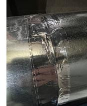
Ensure there is an airtight connection between the supply duct and each CB-SH duct connection. Duct connections should meet SMACNA class B standard up to 2 in. W.G. Refer to Division 23 – Heating, Ventilation and Air Conditioning (HVAC) Section 23 31 13.01 "Metal Ducts" and or Section 23 07 13 "Duct Insulation" for additional information.
