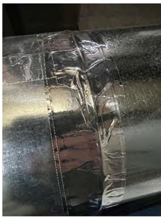
Ensure there is an airtight connection between the supply duct and each CS-ID duct connection. Duct connections should meet SMACNA class B standard up to 2 in. W.G. Refer to Division 23 – Heating, Ventilation and Air Conditioning (HVAC) Section 23 31 13.01 “Metal Ducts” and or Section 23 07 13 “Duct Insulation” for additional information.
